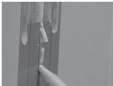
FIGURE 19: BUMP ADHESIVE IN TO PREVIOUS SECTION
