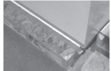
FIGURE 22: HORIZONTAL SEAM FILLED COMPLETELY WITH SEALANT
