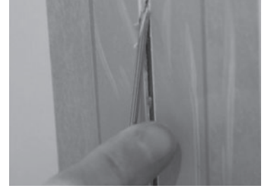
FIGURE 12: REMOVE EXCESS ADHESIVE
