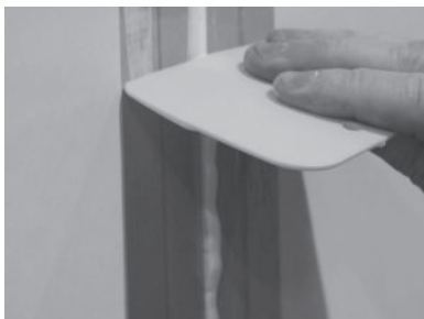
FIGURE 18: REMOVING EXCESS SEALANT
