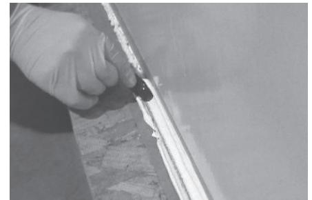
FIGURA 23: HORIZONTAL FINISH WITH ROUNDED CORNER
