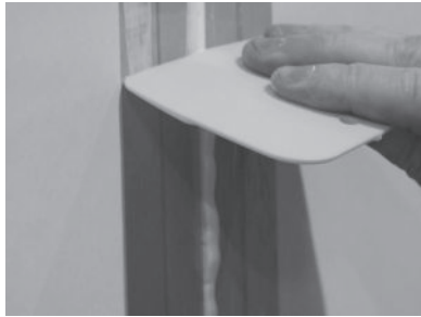
FIGURA 18: REMOVING EXCESS SEALANT
