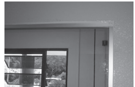
FIGURA 24: TYPICAL WINDOW SEAM APPLICATION
