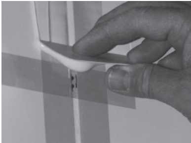
FIGURA 17: APPLYING THE PAINTER TAPE HORIZONTAL IN 3' SECTIONS
