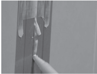
FIGURA 19: BUMP ADHESIVE INTO PREVIOUS SECTION
