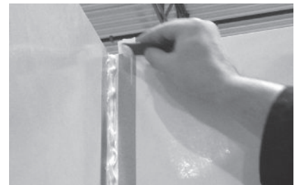
FIGURA 21: USING RADIAL SEAM FINISHER FOR ROUNDER CORNER JOINT
